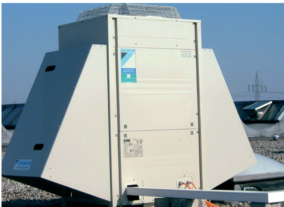
Installation site of the ZEAS with weather protection
