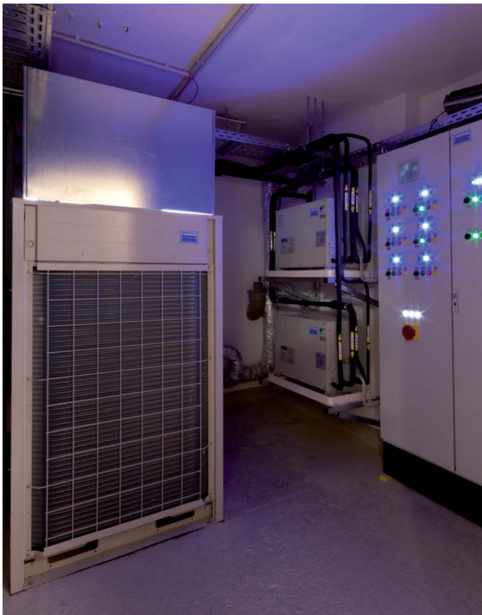
Installation location for the ZEAS and the two boosters
